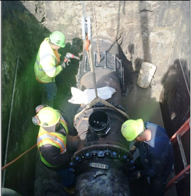
A Distribution Division field crew installing a new fire hydrant connection on a 24" diameter water main, to improve the City's ability to clean and test this main.
